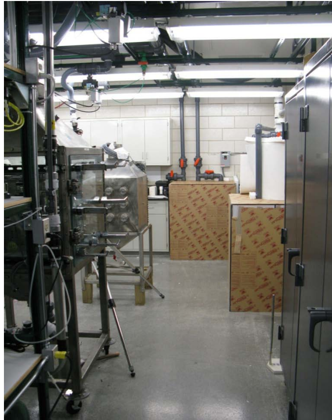
Figure 12. View of acoustical enclosures surrounding air compressors
